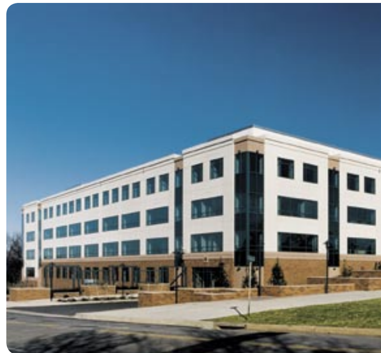
The LEED-certified Social Security Annex building in Baltimore, MD features an HVAC system that utilizes Victaulic products.
